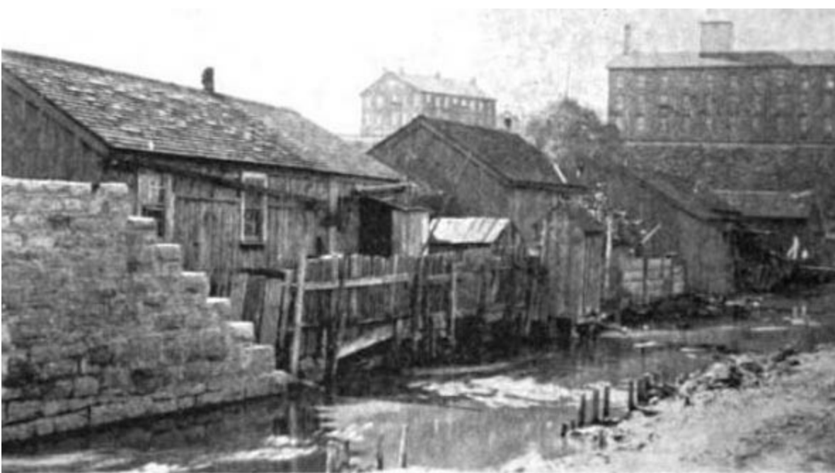
Photo 1.1: Syracuse, NY—Shanties Back to an Open Sewer. (1901)
