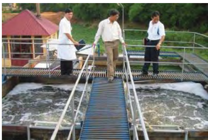
Figure 9.3 Activated sludge wastewater-treatment system in a hospital in Sonla, Vietnam
